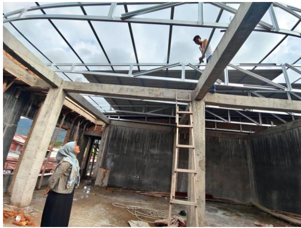
Figure 3. Field roof truss installation.
