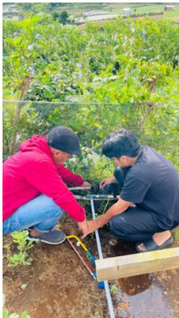
Figure 3. Installation of Irrigation Pipes, Soil Moisture Sensor
